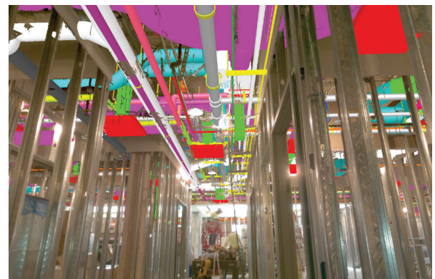
3D laser scan model displaying planned MEP for Houston Methodist Sugar Land Hospital, Sweetwater South Expansion and Renovation
