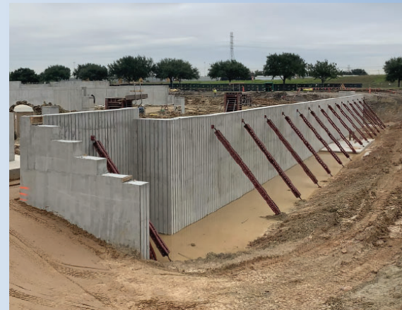
Pond retention wall at the University of Houston, Garage Number 6
